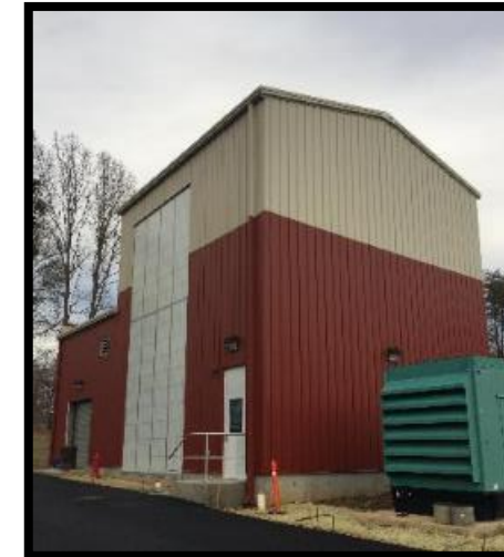
North Rivanna WTP
