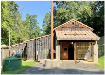
1 EXISTING CONDITIONS PHOTO FRONT OF PS3
