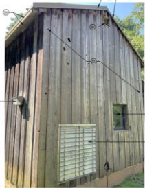
4 EXISTING CONDITIONS PHOTO BASIN SIDE OF PS3
