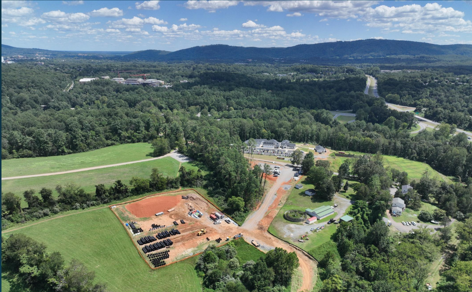
Ragged Mountain RWPS and Pipeline
