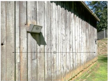
3 EXISTING CONDITIONS PHOTO FRONT OF PS3
