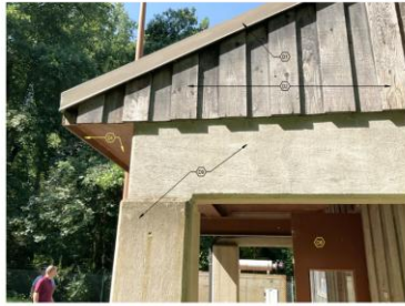
2 EXISTING CONDITIONS PHOTO BASIN SIDE OF PS3
