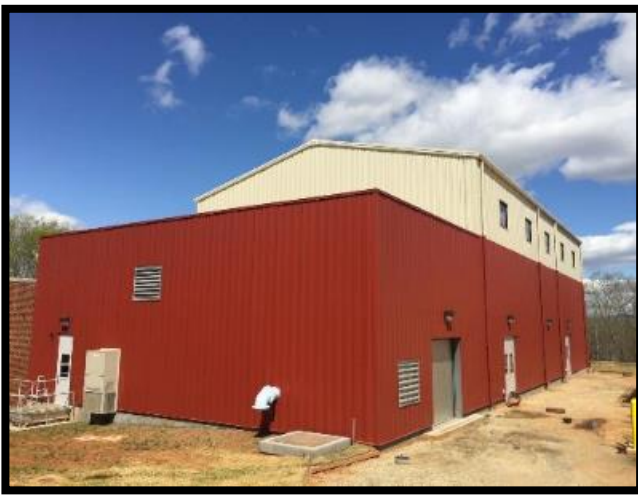
South Rivanna WTP
